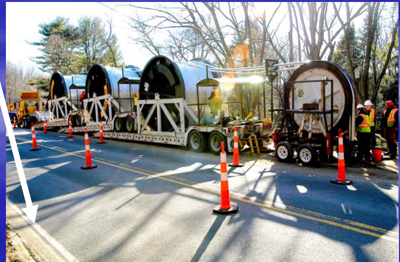
3 cable underground pull
