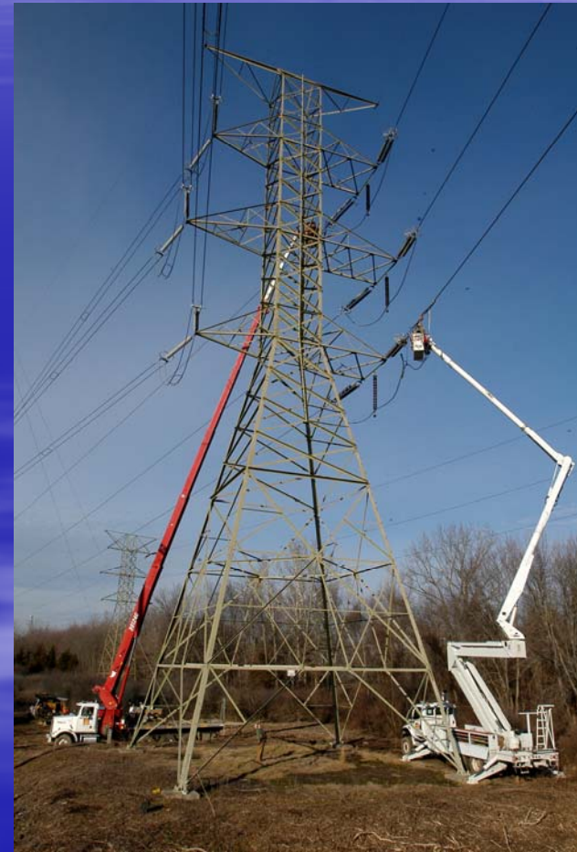
Electrical maintenance using aerial lifts
