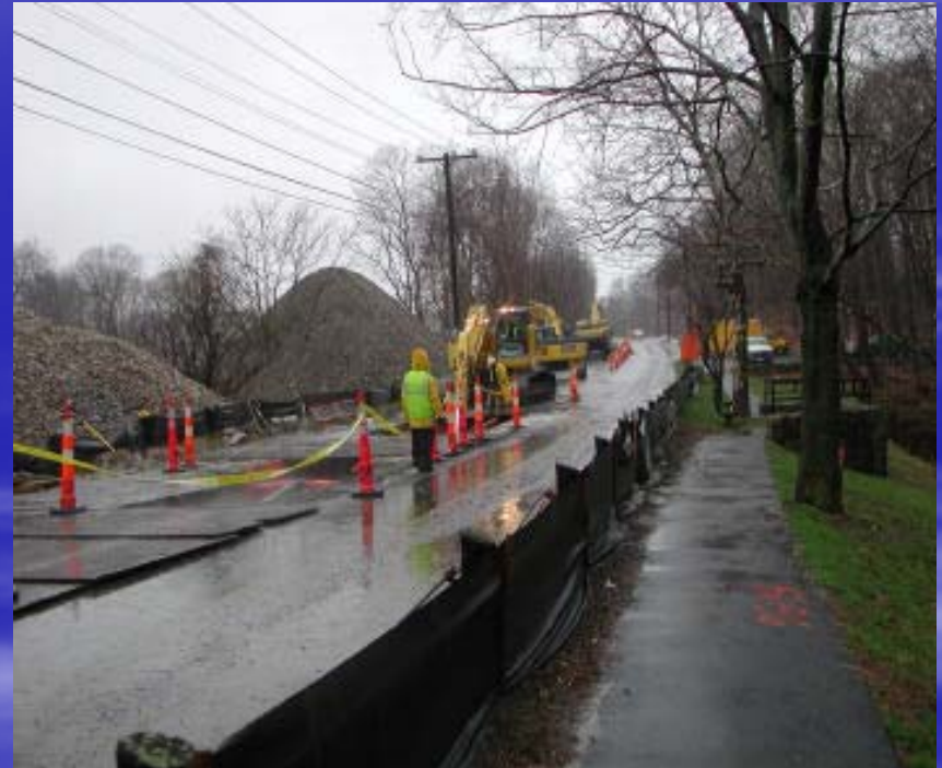
Trenching with tracked excavators
