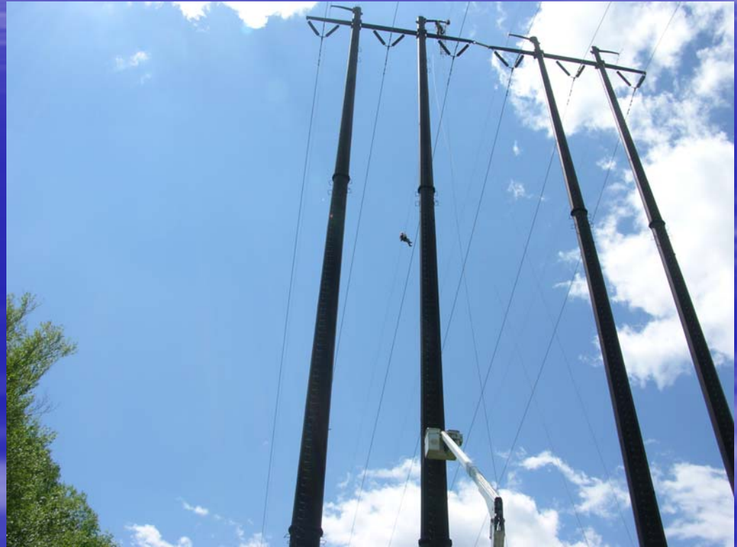
Work positioning from transmission line structure cross arm maintenance
