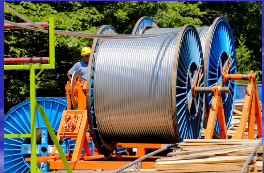
Wire stringing operation
