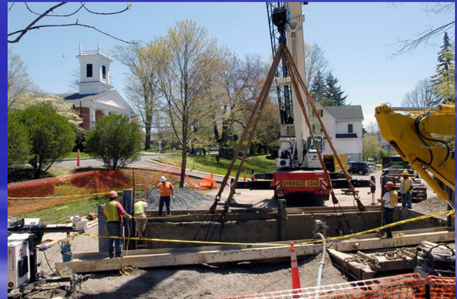
Installation of an underground electrical vault
