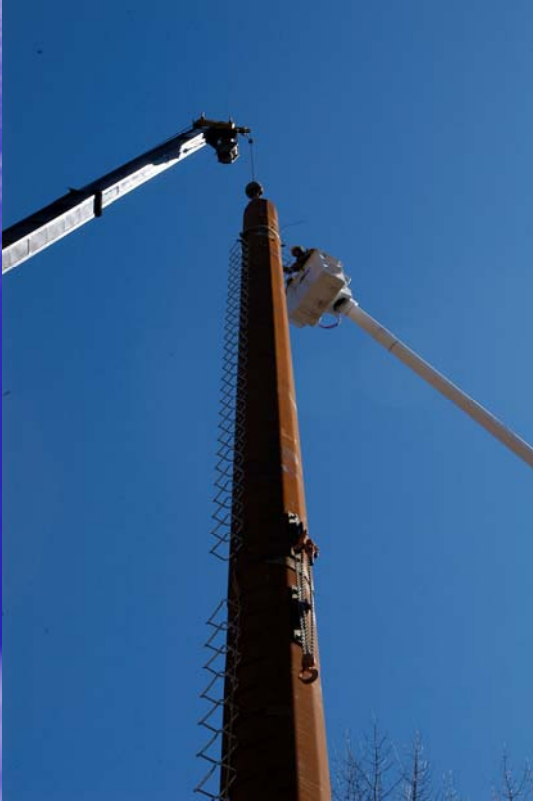
Construction of mono poles
