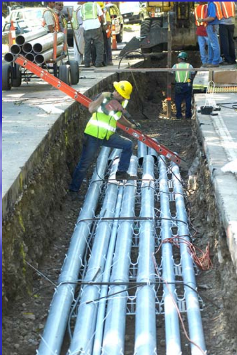
Underground transmission cable installation
