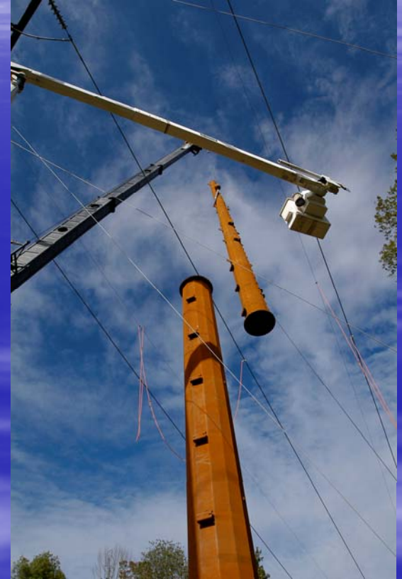
Construction of mono poles
