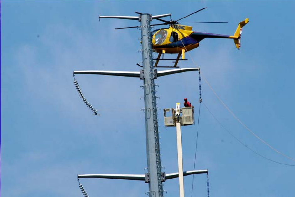
Wire stringing via helicopter
