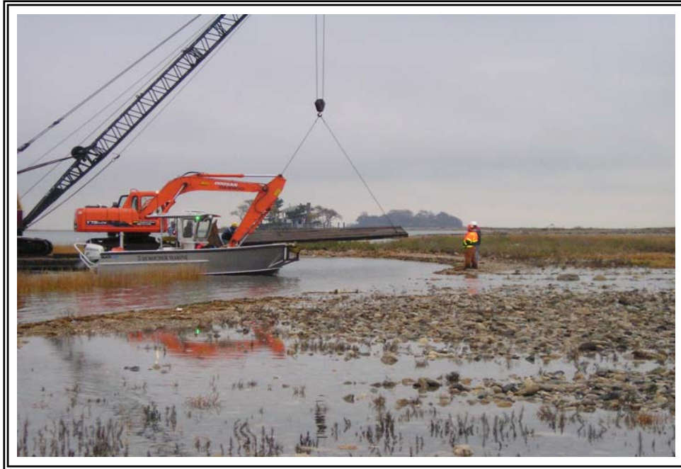
Photo 3: Equipment mobilization onto Sheffield Island, avoiding existing Spartina .
